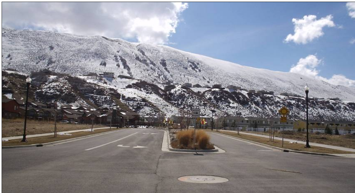
Traffic Calming, Center Island, 65 East, south of Highland Drive
