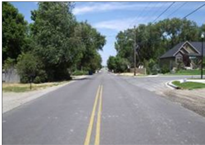
300 East at 13700 South looking north
